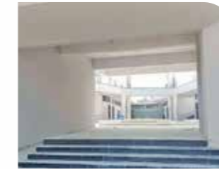
Construction of 'We Care Nursing School' at Surat, Gujrat.
