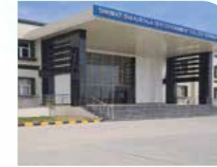
Construction of 'Smt. Shakuntla Devi College' at Sidhmukh, Churu, Rajasthan.
