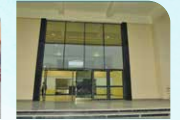
Maintenance of 'Smt. Mohini Devi Chachan Govt. College', Sahawa, Churu, Rajasthan.
