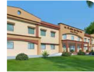
Construction of 'Shri Manoj Gupta Govt. Senior Secondary School' at Sidhmukh, Churu, Rajasthan.
