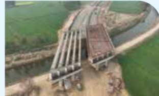
Yamuna Bridge Highway (HAM)
