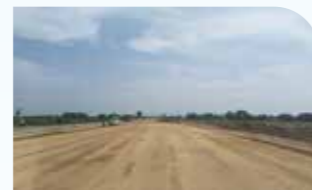
Kasganj Bypass (HAM)
