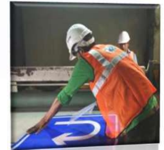
ROAD SIGNAGES, CONSTRUCTION CHEMICALS AND MARKING PAINT
