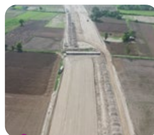
Kasganj Bypass (HAM)
