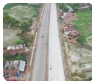
Yamuna Bridge Highway (HAM)
