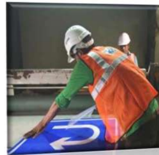
ROAD SIGNAGES AND MARKING PAINT
